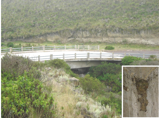
Figure 1. Panoramic view of Jatunhaico creek canyon and bridge, Reserva Ecológica Antisana, Pichincha-Napo, Ecuador. Inset: one of the eleven nests of Ecuadorian Hillstar ( Oreotrochilus chimborazo ) found in the underside of the bridge in 2007. Photo: A. Solano-Ugalde
